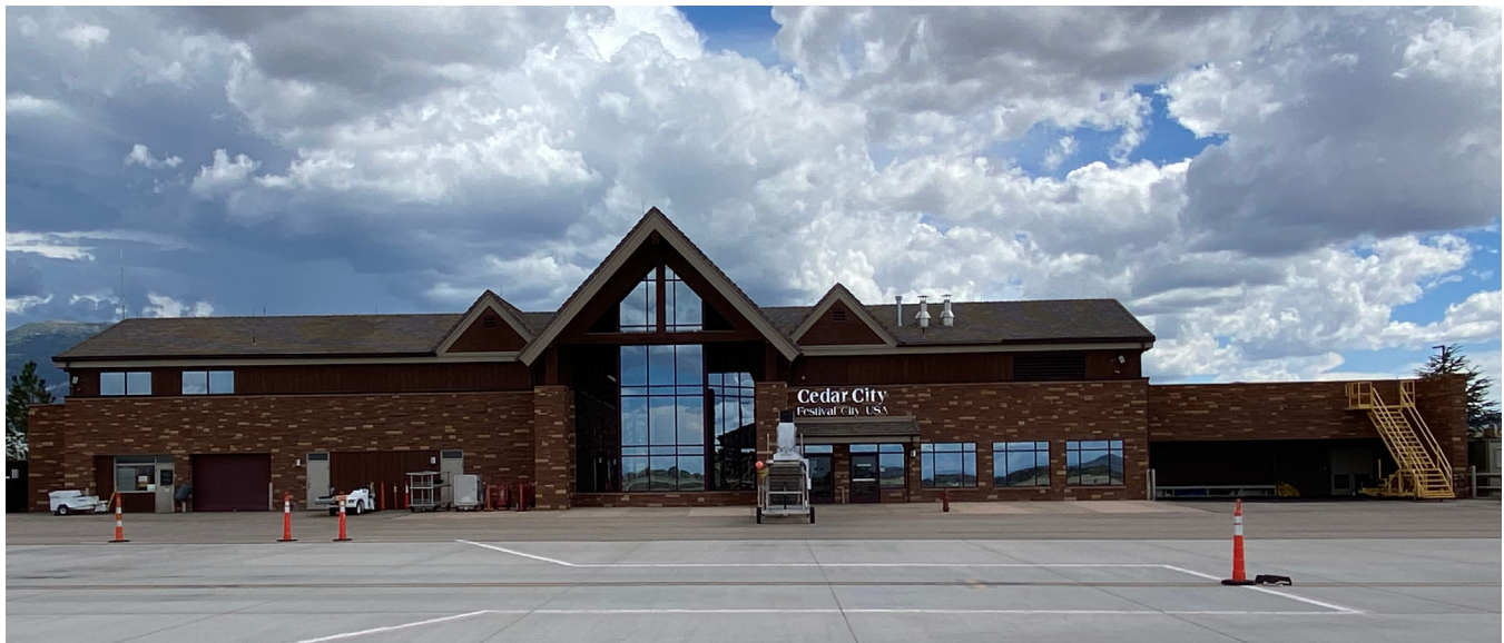
Figure 4.20: Passenger Terminal Building
