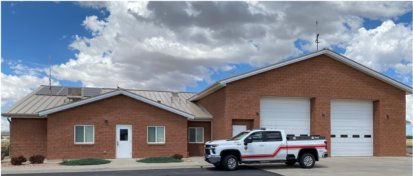
Figure 4.33: Cedar City Fire Station #3
