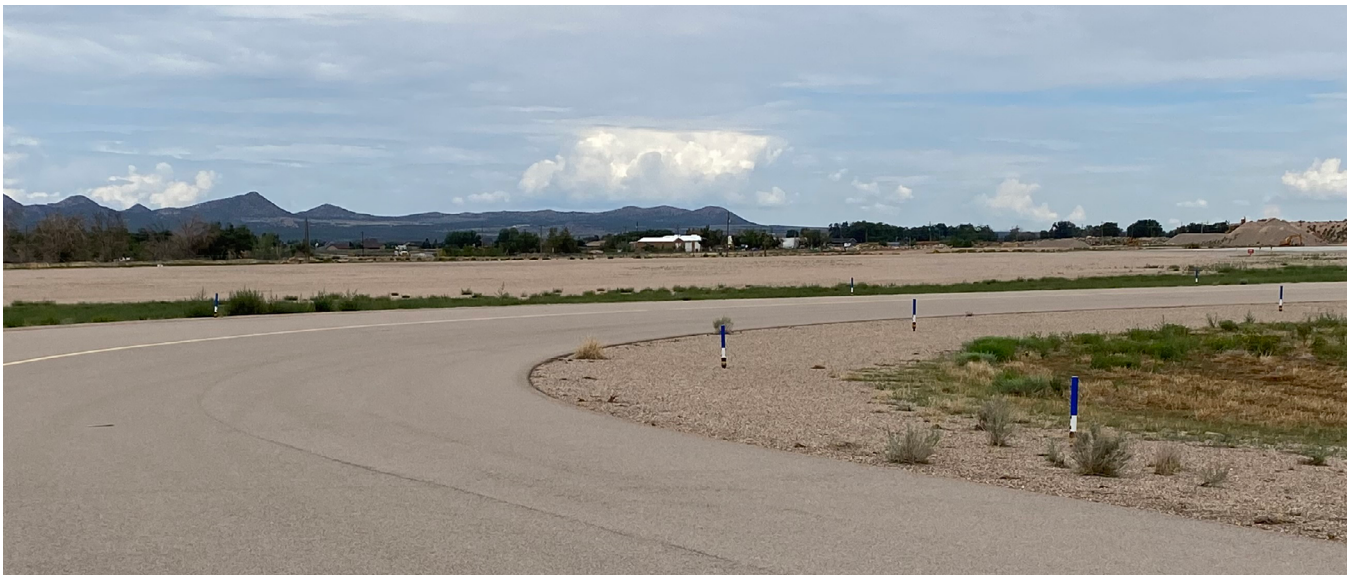
Figure 4.15: Taxiway Edge Reflectors
