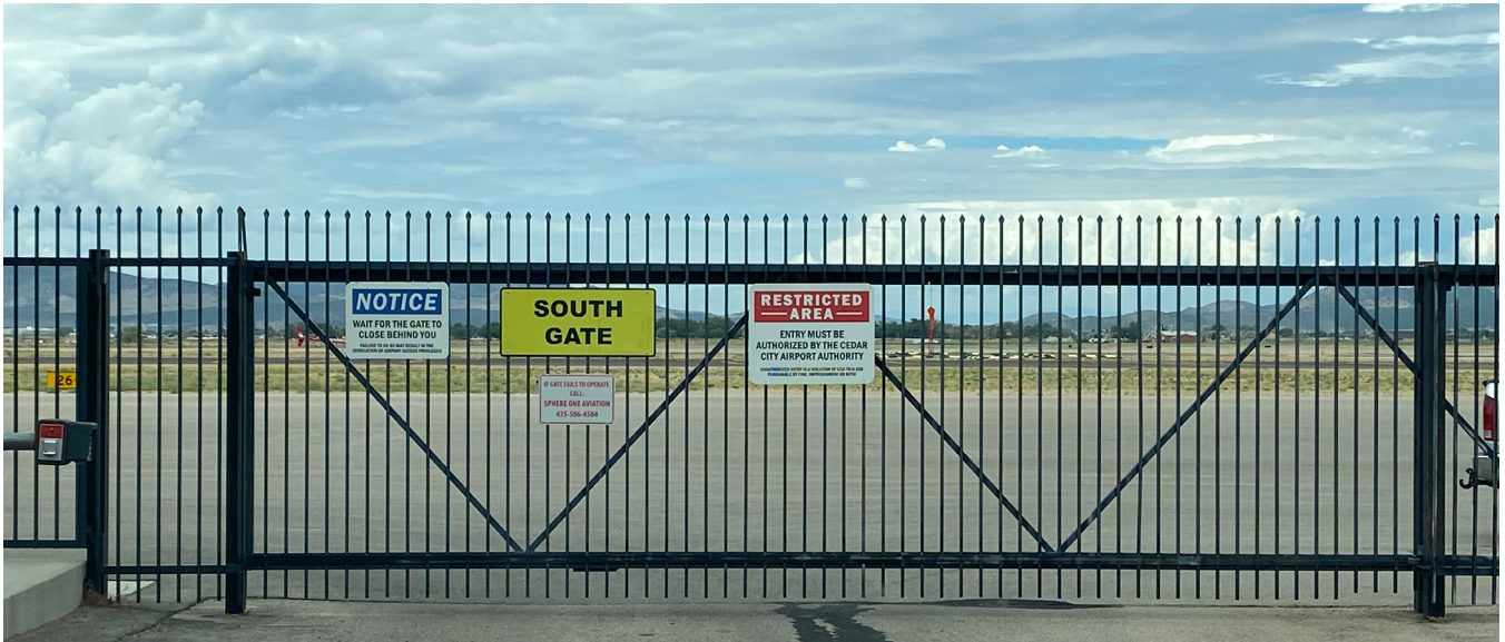
Figure 4.37: Vehicle Security Gate
