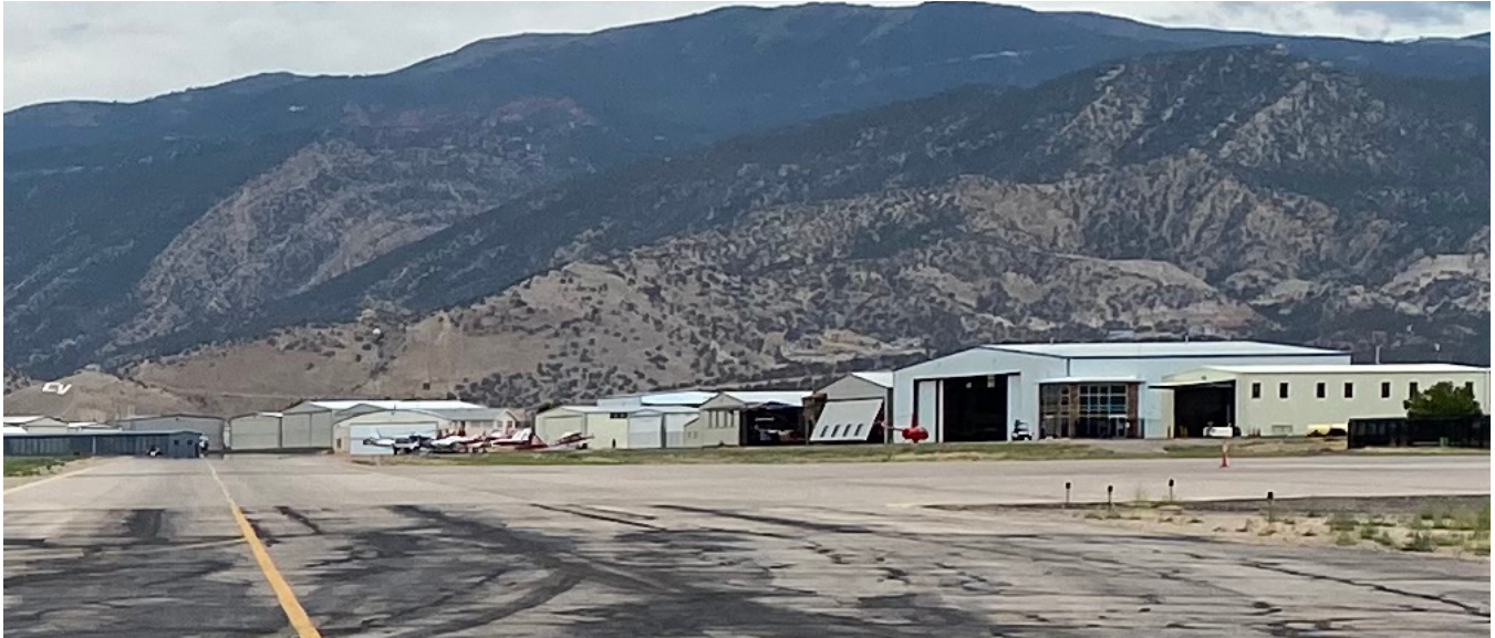
Figure 4.28: Main Hangar Area
