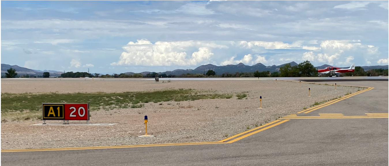
Figure 4.14: Medium Intensity Taxiway Lights
