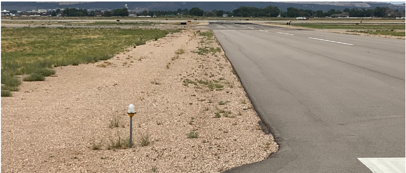
Figure 4.13: Runway Edge Lighting
