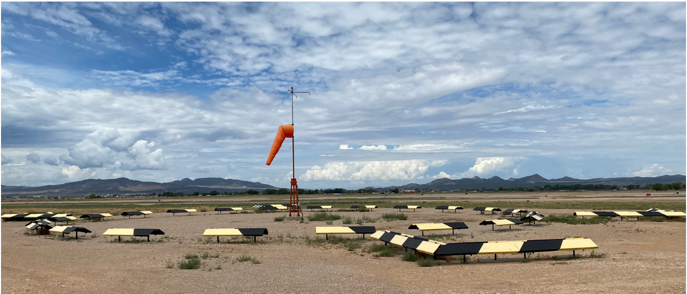
Figure 4.17: Segmented Circle and Wind Indicator
